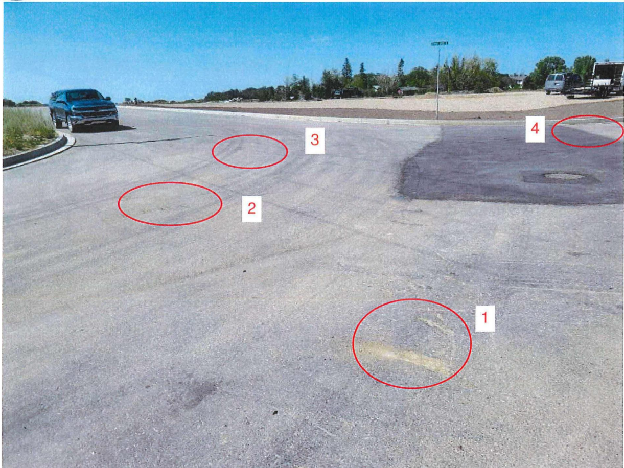
Figure 3: Locations of the 4 existing asphalt damages due to equipment.
