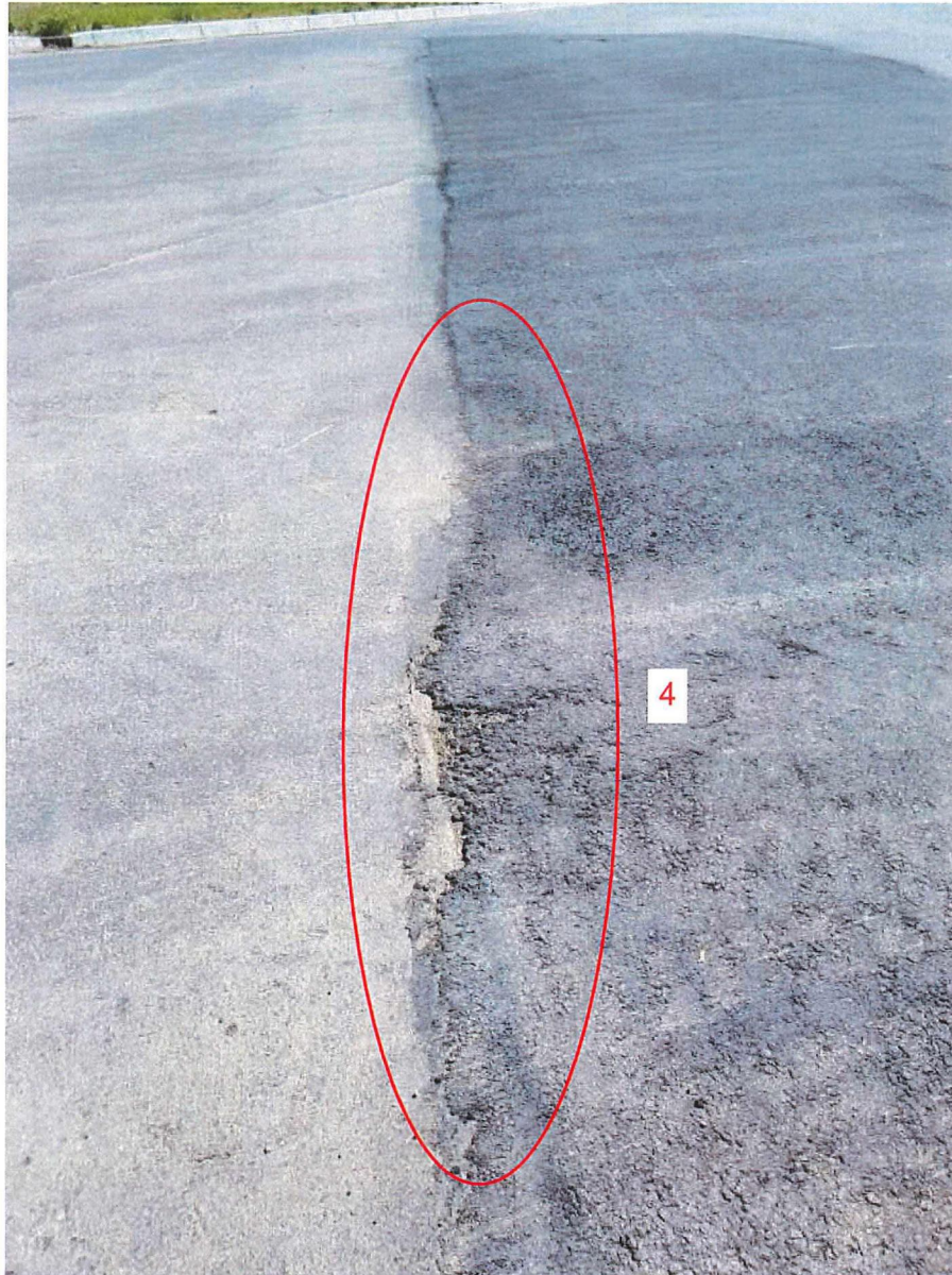
Figure 6: Locations of the existing asphalt damages due to equipment.
