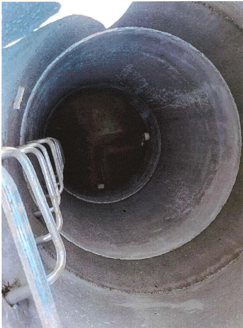
Figure 1: Gravel in sanitary sewer service line manhole.
