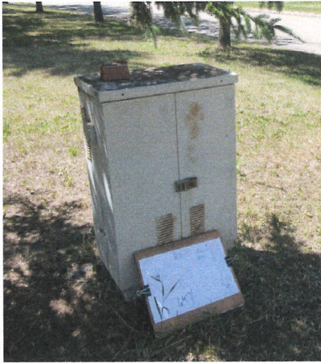
Pedestal to be replaced
